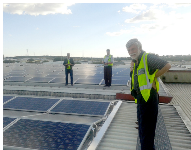
Visiting the largest rooftop PV installation (09.05.2014 - Windhoek, Namibia)
